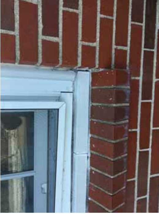
Figure 25: Exterior window caulk
