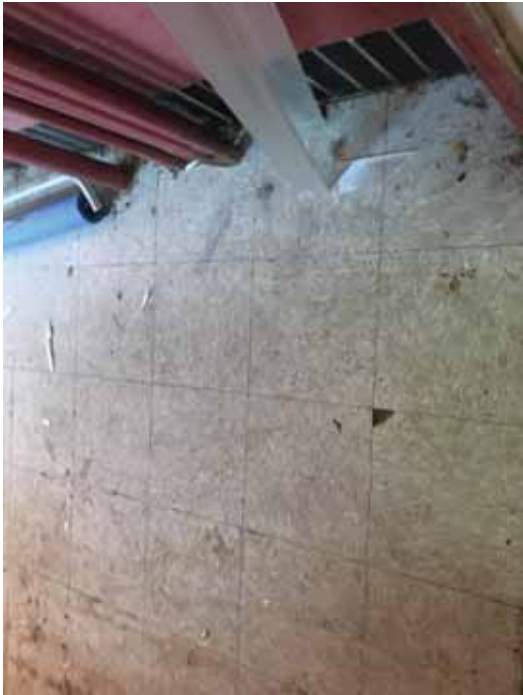
Figure 22: 12" x 12" Grey mottled floor tile (underlain by ACM mastic)
