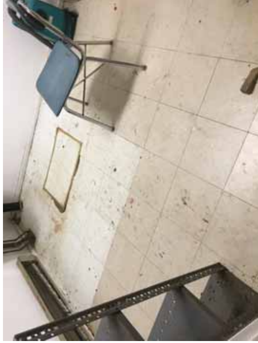
Figure 12: 12" x 12" White with multicolor fleck floor tile
