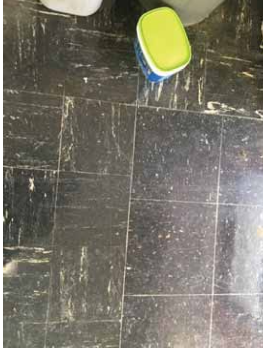
Figure 20: 12" x 12" Black streak floor tile (bottom left). Remaining floor tile is ACM 9"x9" Black streak floor tile.
