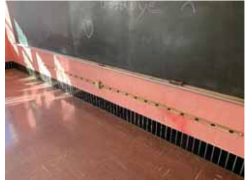
5.9: Outlets installed using surface raceway
