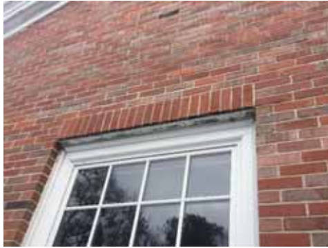
2.12: Typical condition of steel lintel at window
