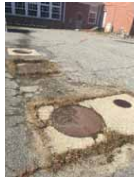
1.3: Underground fuel storage tank
