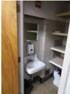
3.8: Remove fixtures in storage closet
