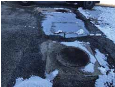
4.7: Parking Lot – Fuel oil tank access covers
