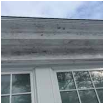
2.2: Scrape and paint soffit, rake and eave trim throughout
