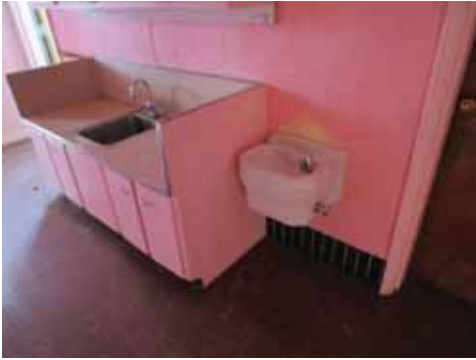
3.17: Typical classroom sink and casework
