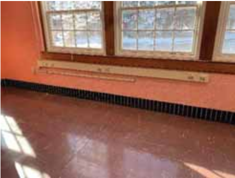
5.10: Outlets installed using surface raceway
