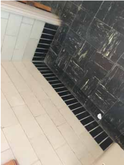
Figure 13: ACM 9" x 9" Black streak floor tile (mastic is non-asbestos)
