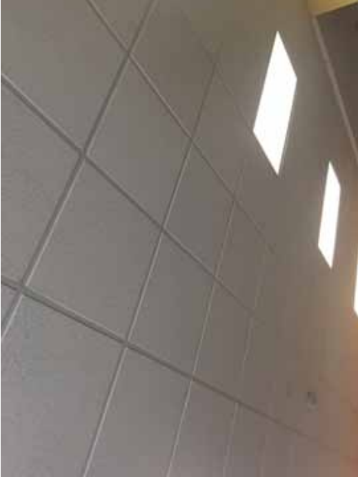
Figure 19: 2' x 2' Crow feet ceiling tile
