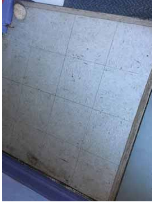
Figure 10: 12" x 12" White with blue streak floor tile
