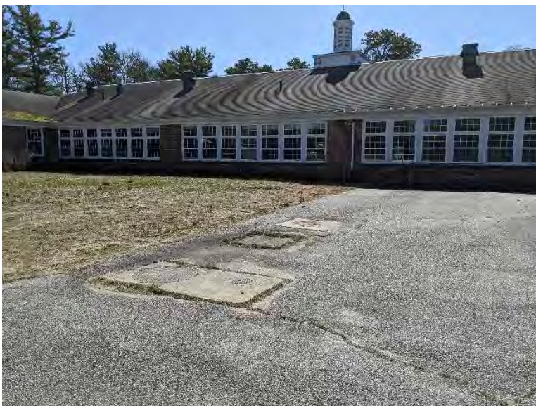
Photo 1: Former location of UST behind school building, prior to removal.
