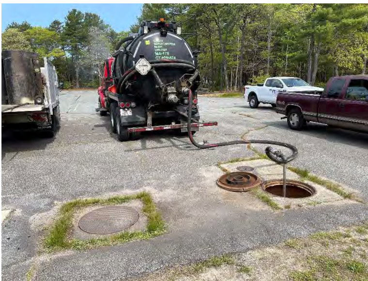
Photo 2: Boston Green pumping out majority of tank contents on May 15, 2023.
