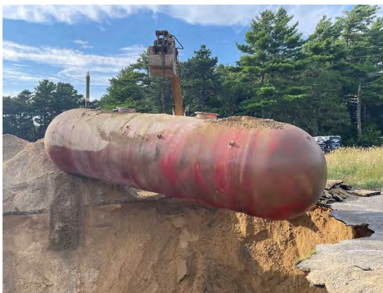
Photo 4: UST after being removed from the ground.
